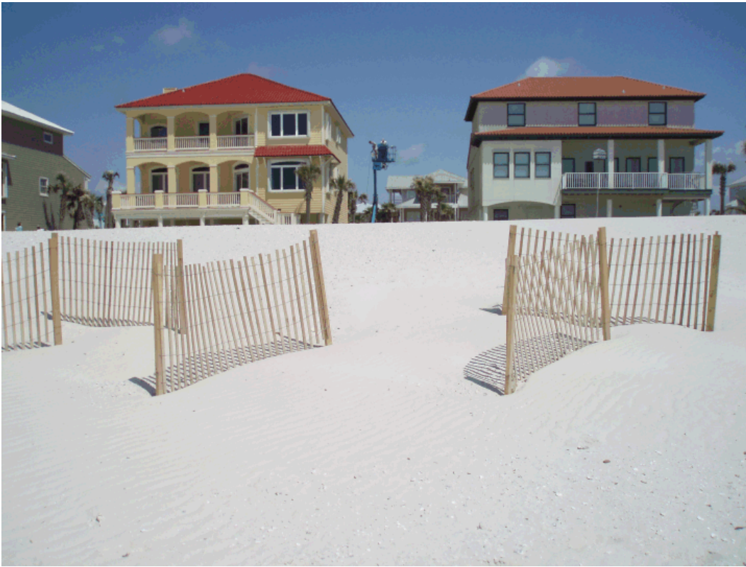
Accumulation of several inches depth of sand behind private sand fencing
