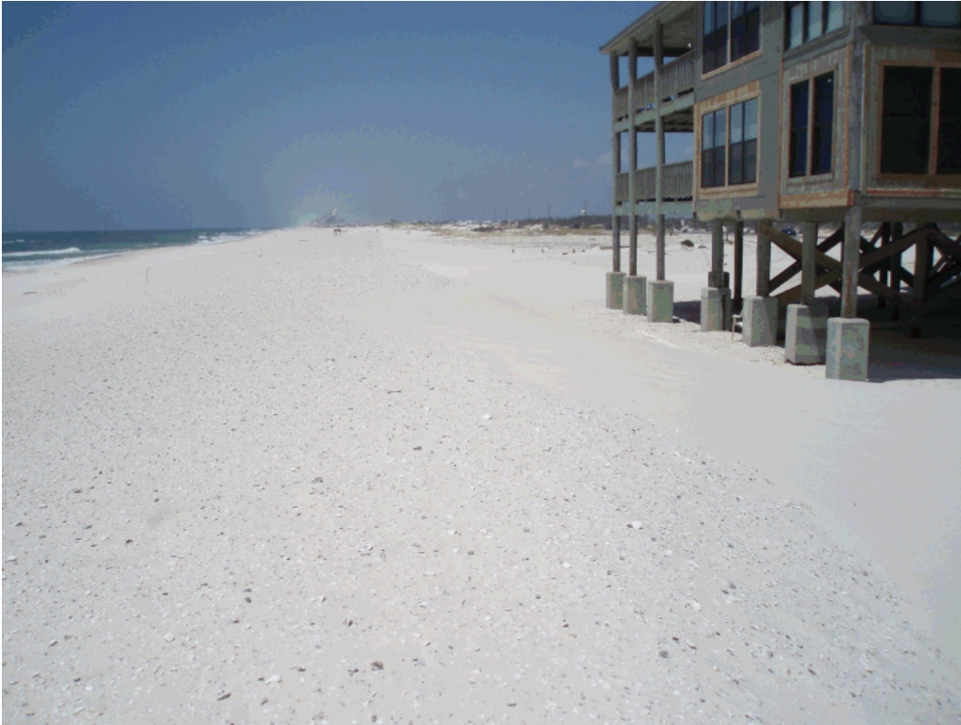
Reduced deposition behind dune directly in front of structure, and increased deposition in lee.
