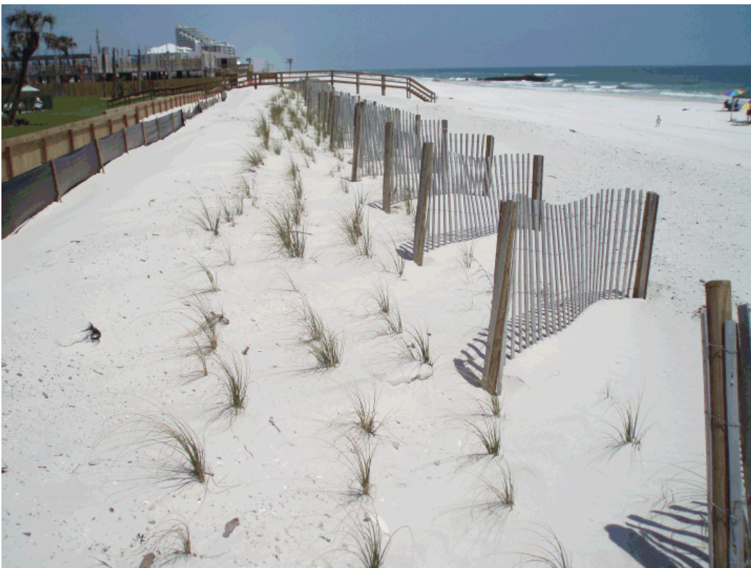
Relatively modest accumulation by sand fences, due to alignment with wind direction.
