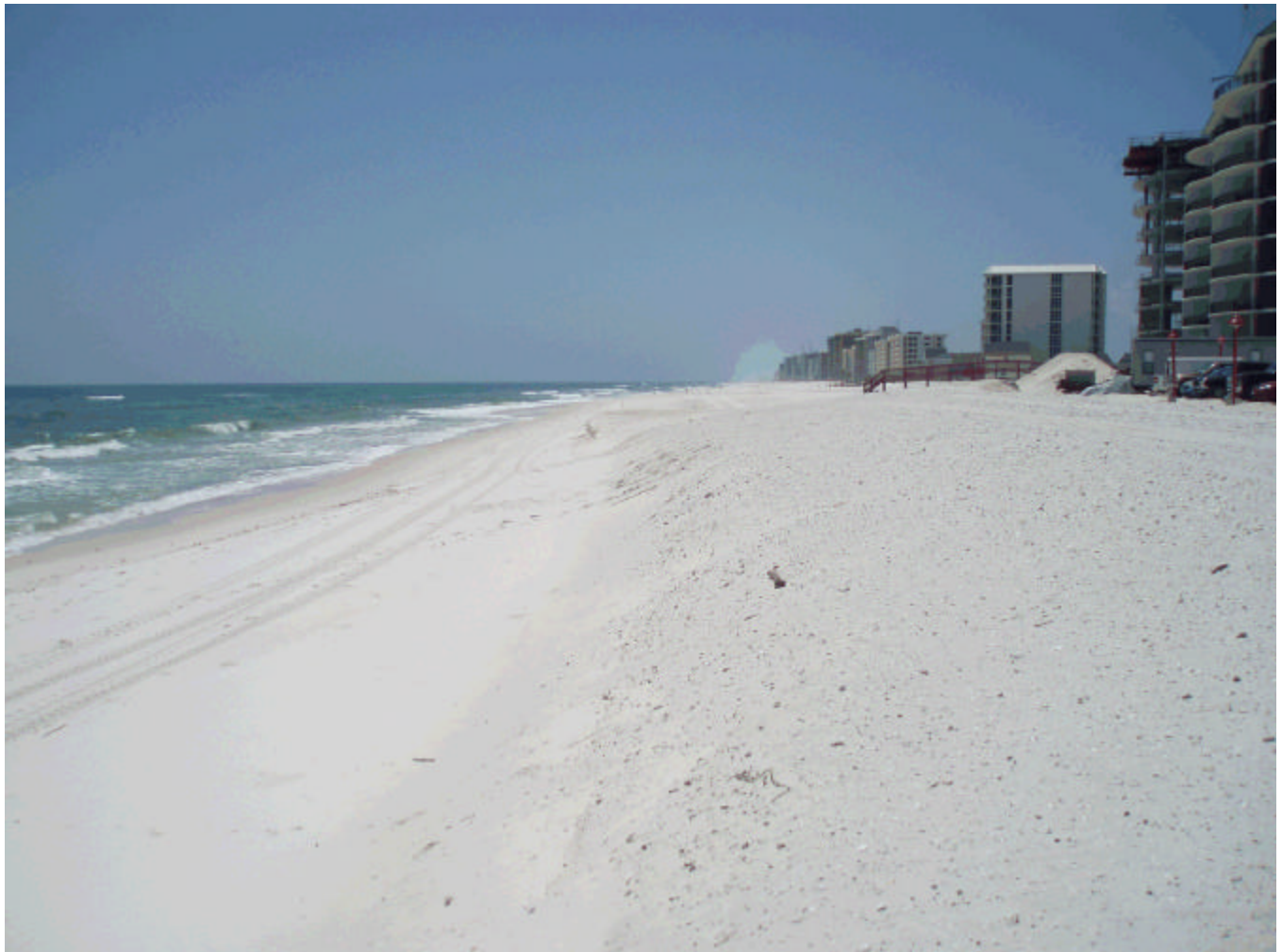
Erosion scarp on dune face behind the Crab Trap Restaurant, observed on March 2, 2006
