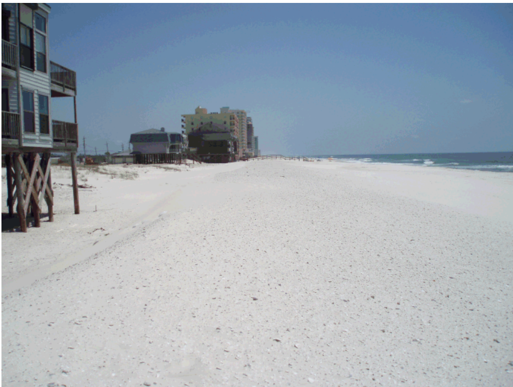
Reduced deposition behind dune on windward side of structure.
