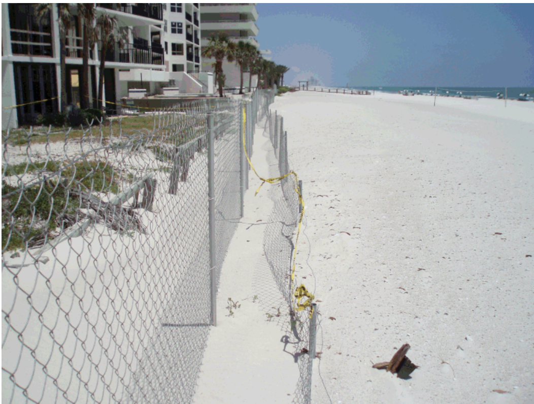
Good illustration of quantity of sand accumulated behind dune. Note relative modest burial of grass behind fence.
