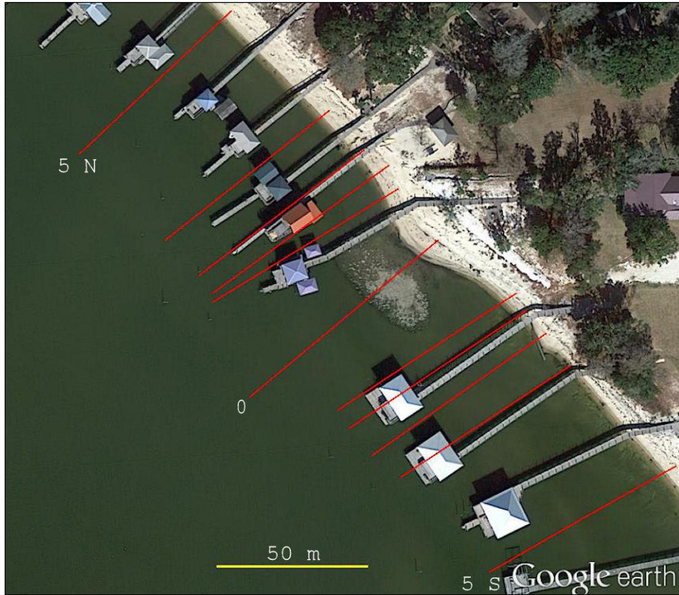
Figure 4. Project post construction, 1/30/2015, with survey profiles 5S through 5N
